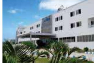
Rudrapur Plant (Green Building)
